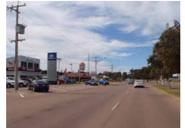
PHOTO 8 - RELATIVELY WIDE ROAD RESERVES THROUGHOUT THE TOWN CREATE UNCONTAINED STREETSCAPES THAT REFLECT A SENSE OF SPACIOUSNESS
