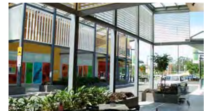
PHOTO 22 - LOCAL CLIMATE CONTROL THROUGH CLEVER DESIGN OF BOTH PUBLIC AND PRIVATE REALM
