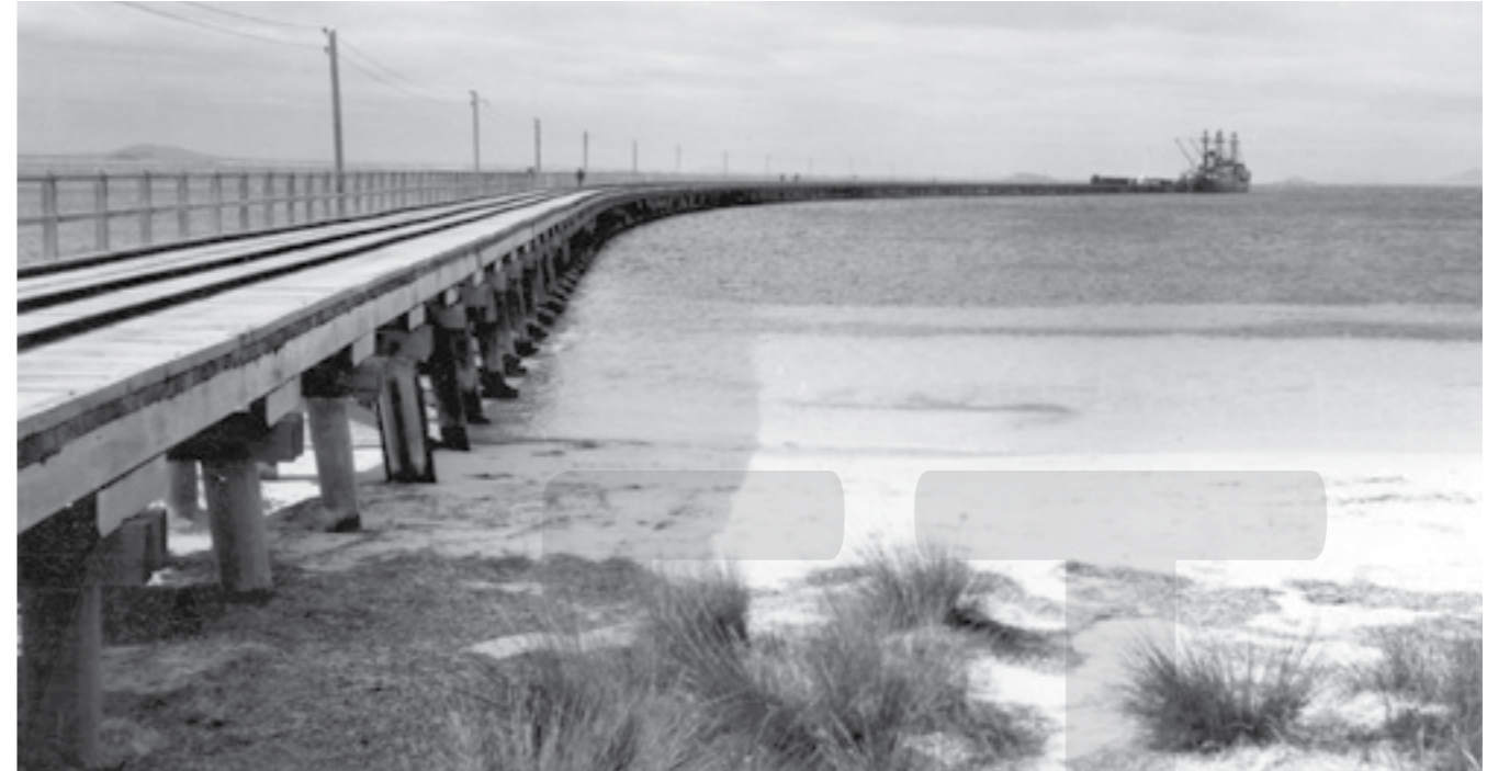
PHOTO 2 - TANKER JETTY, 1955 (SOURCE: BATTYE LIBRARY)
