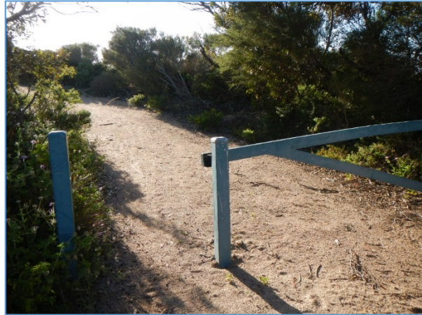
Figure 18 Steel gateway installed on the Lovers Cove track
