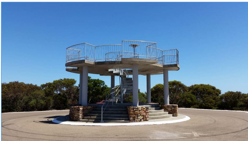
Figure 14 Current Rotary Lookout following refurbishment in 2017 (view south)
