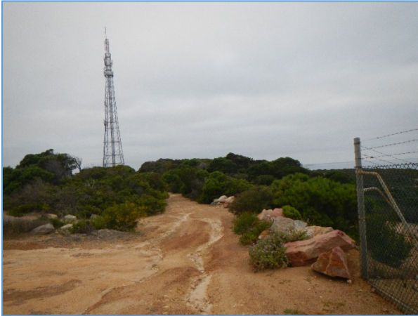
Figure 17 View north east along track to the telecommunications tower
