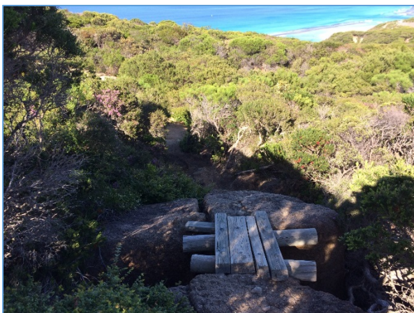
Figure 38 Unauthorised structure present on western side of Dempster Head
