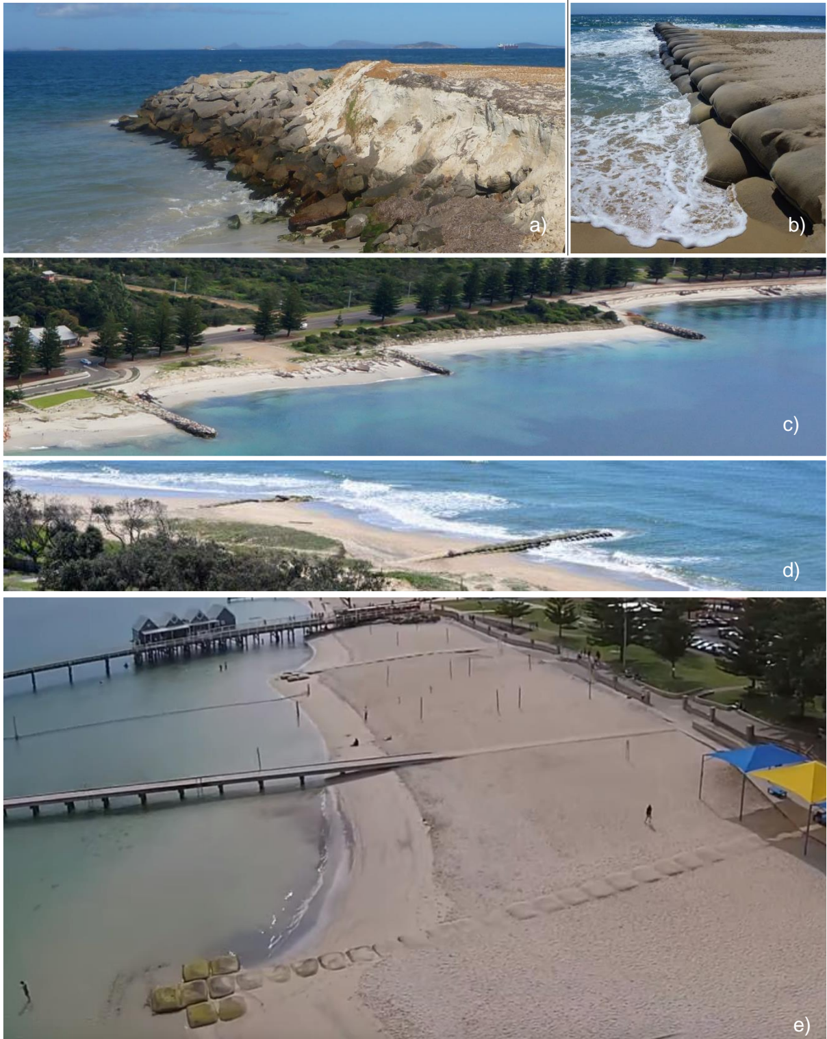
Figure 3-11: Illustration of groyne options: Rubble-mound groynes Esperance Norseman Rd, WA (a,c); Geotextile groynes: Busselton, WA (e) Maroochydore, QLD (b,d). Photo credit: Hilary Darmody (b,d) and Andrew Mozdzen (d).
