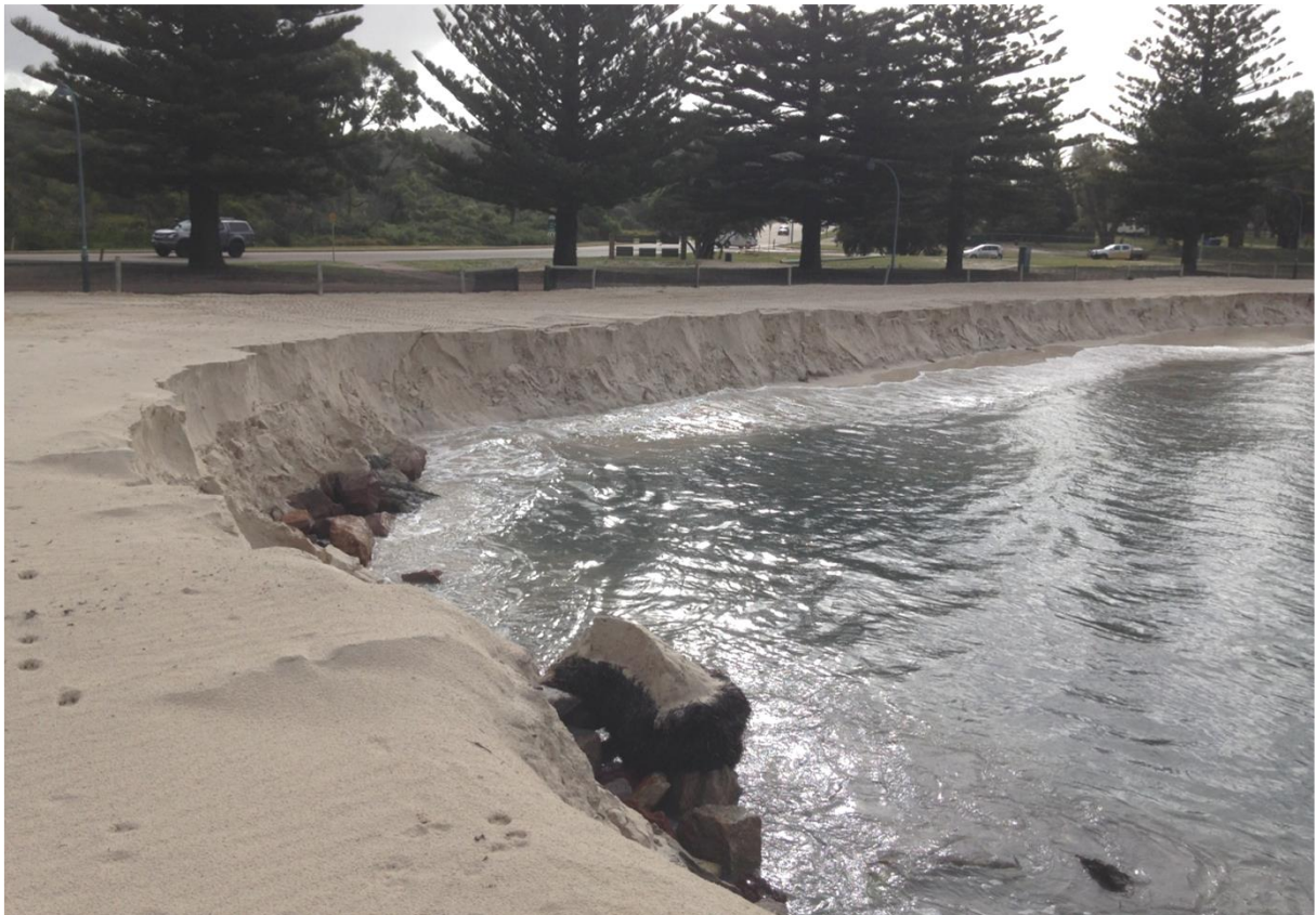
Figure 1-1: Foredune scarp following beach nourishment indicative of high erosion rate at Castletown Beach
