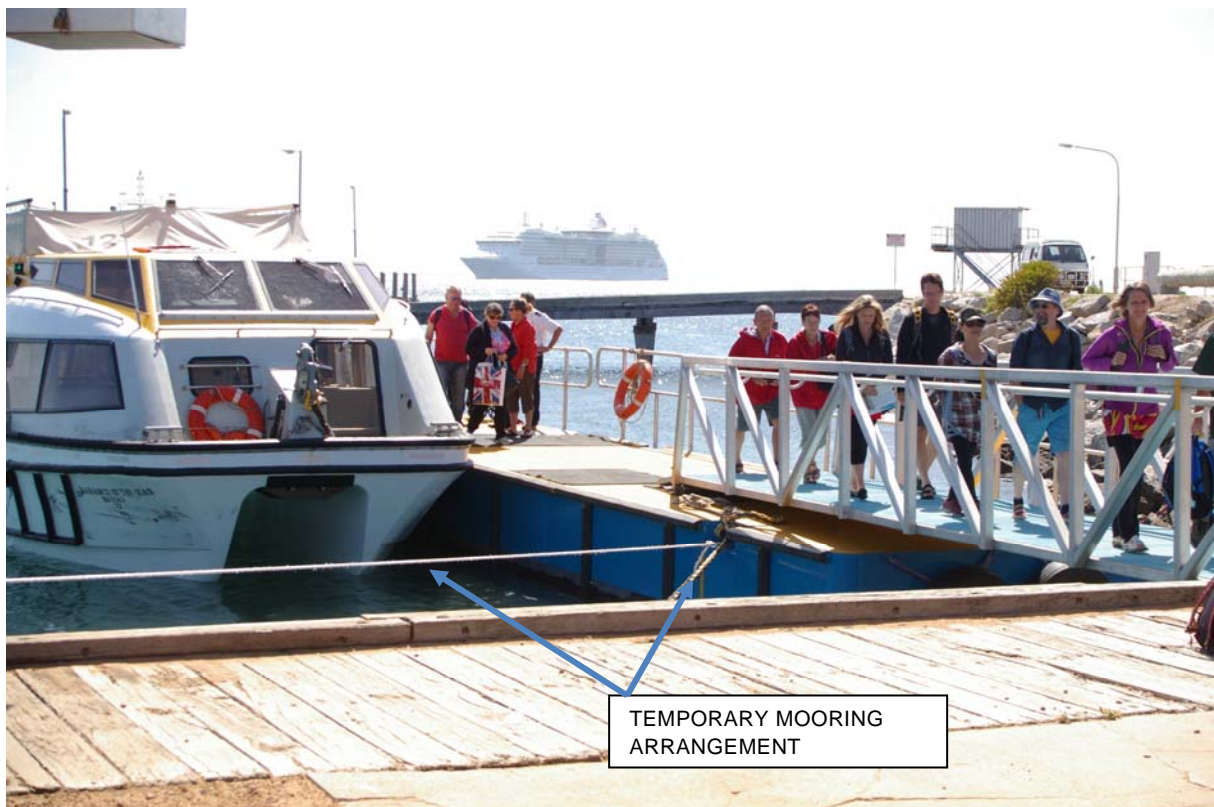
Figure 2.18 Tender Vessel, Pontoon, Gangway and Mooring Arrangement.
