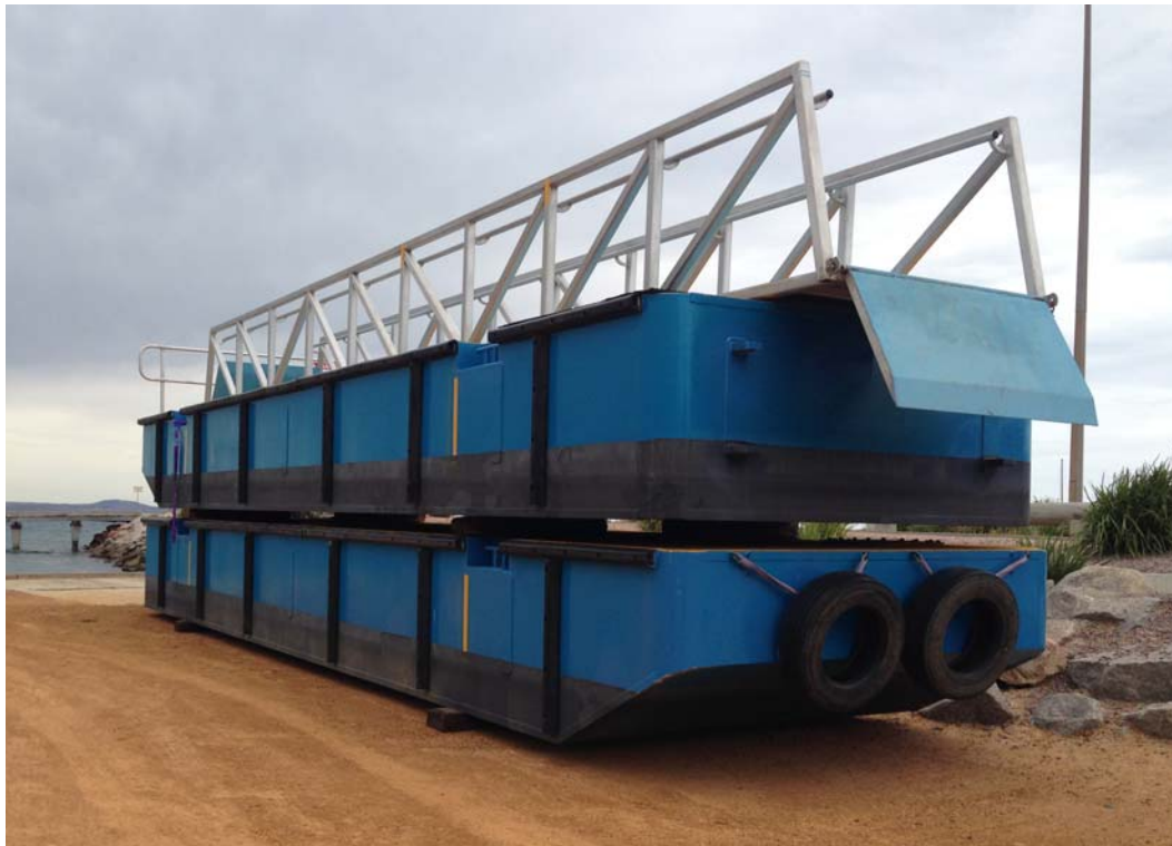
Figure 4.1 Esperance Port Existing Pontoons and Gangway
