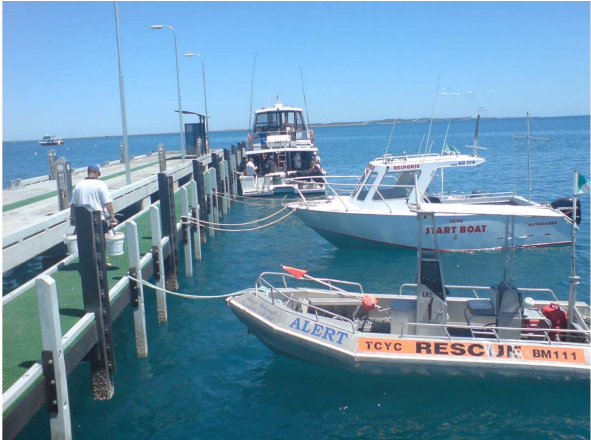
Figure 5.3 Example Fixed Lower Level Vessel Landing
