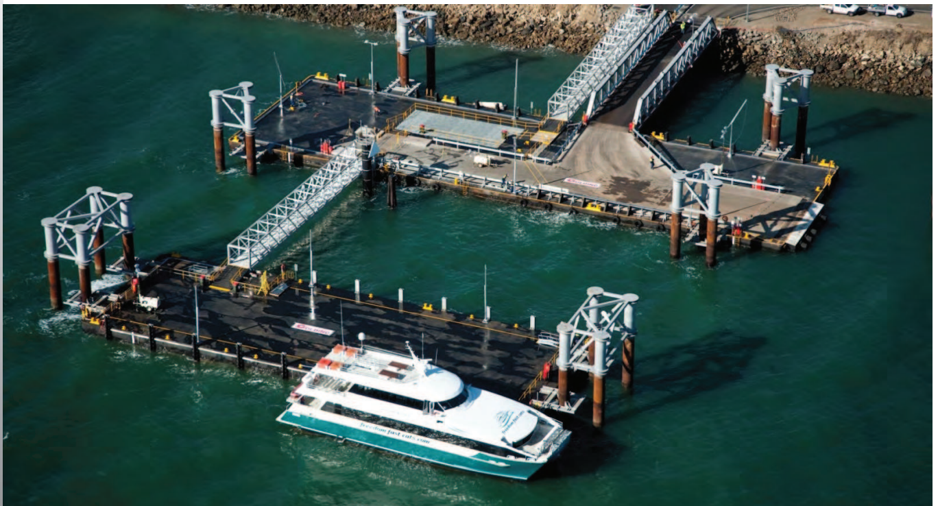
QCLNG – Ferry Dock and Floating RoRo Facility
