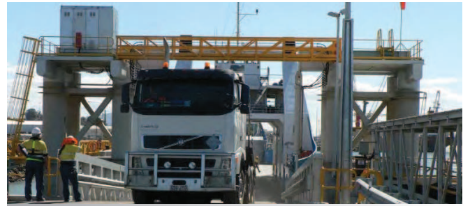
GLNG – Port Central - Linkspan Bridge in operation
