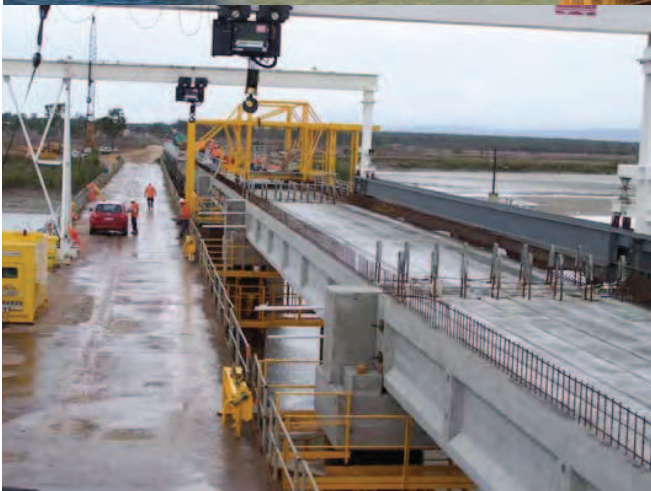
St Lawrence Bridge Duplication
