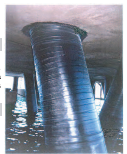
▲ Figure 1. Denso Seashield Series 60 system (excluding Pilemesh) .
