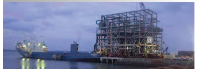
Alcan Gove - Material Offloading Facility (MOF)
