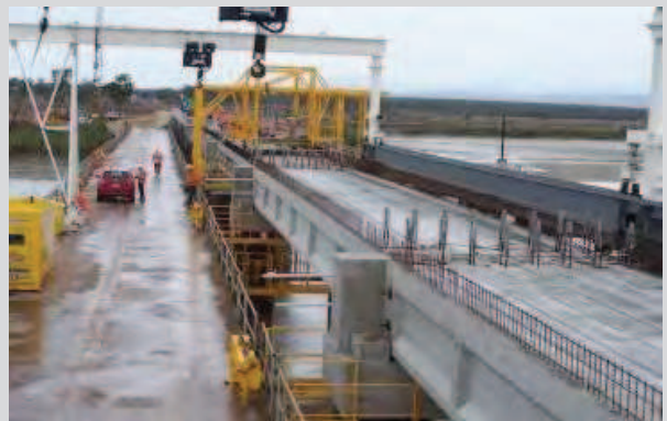
St Lawrence – Rail Bridge Duplication
