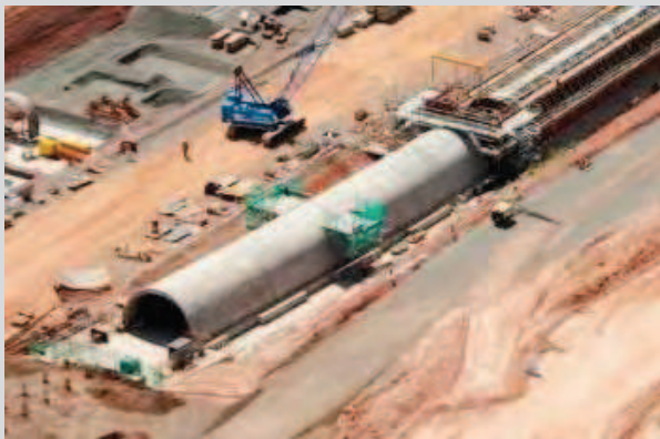
WICET – Reclaim tunnels
