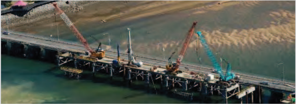
Forgan Bridge – Construction Engineering
