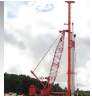
Exxon Mobile – Piling Leader
