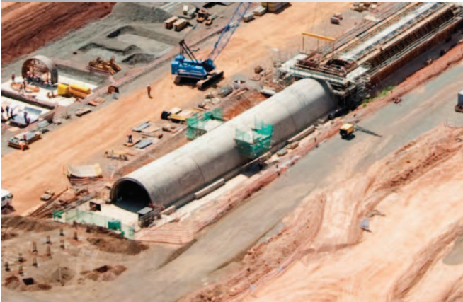
WICET – Coal Reclaim Tunnel
