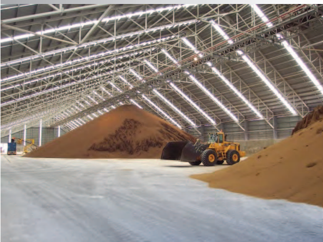
WMC – Fertilizer Stockpile Building
