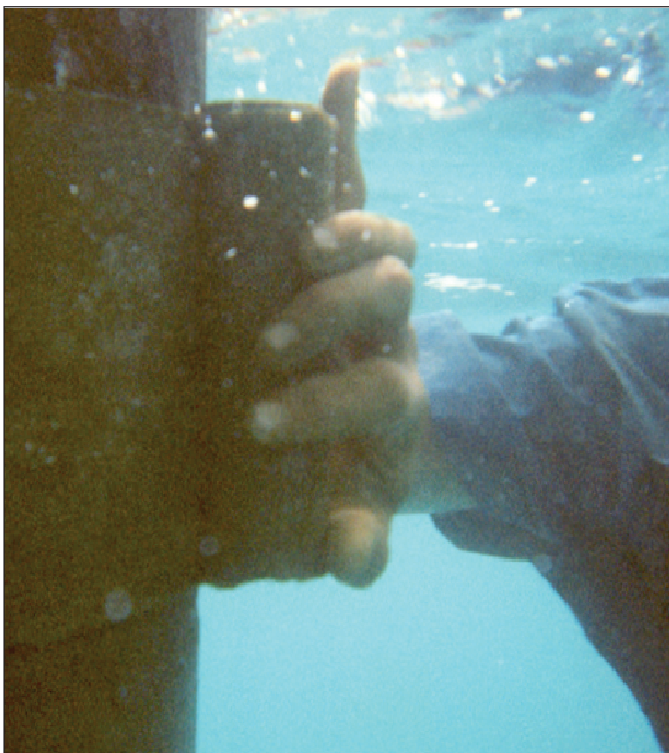
▲ Figure 3. Tape being applied under water.
