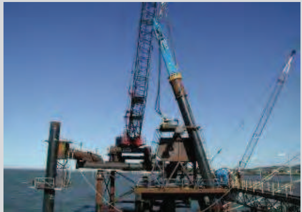
RG Tanna Wharf – Construction Engineering
