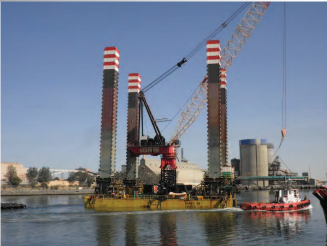
SEP Santa Fe - under tow fitted with Favco Crane
