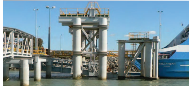
GLNG – Port Central - RoRo Facility c/w hydraulically controlled linkspan bridge.
