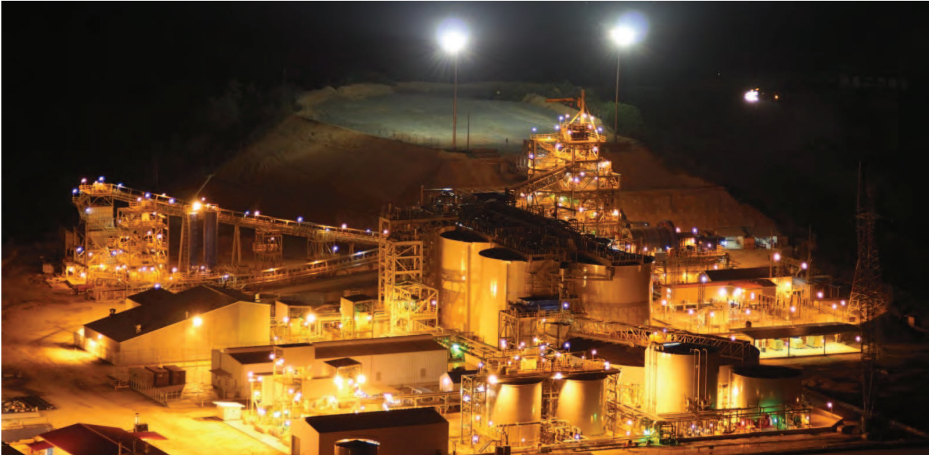
Ban Houayxai - Gold and Silver Plant
