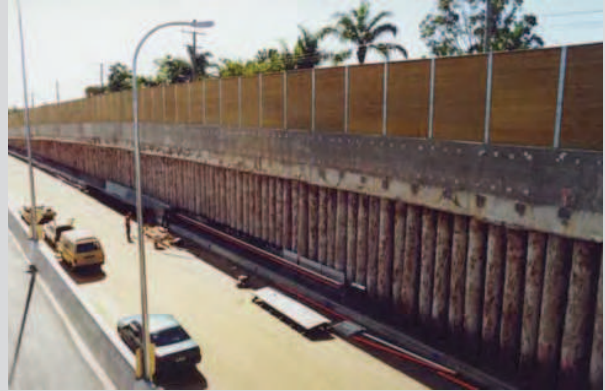
South East Transit Project – Soil Retaining Structures
