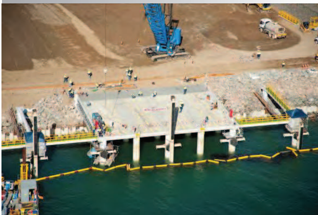
GLNG – RG Tanna - LoLo Facility during construction
