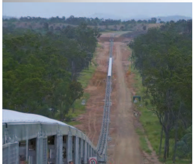
Lake Lindsay – Overland Conveyor
