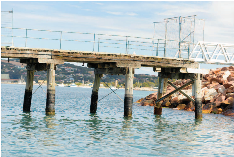
Current aluminium gangway span onto the Jetty
