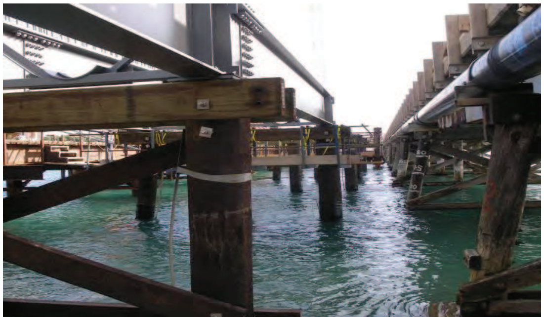
► Figure 2. Timber piles protected in the splash zone.
