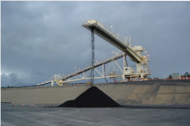
Newpac – Coal Stockpile Basin
