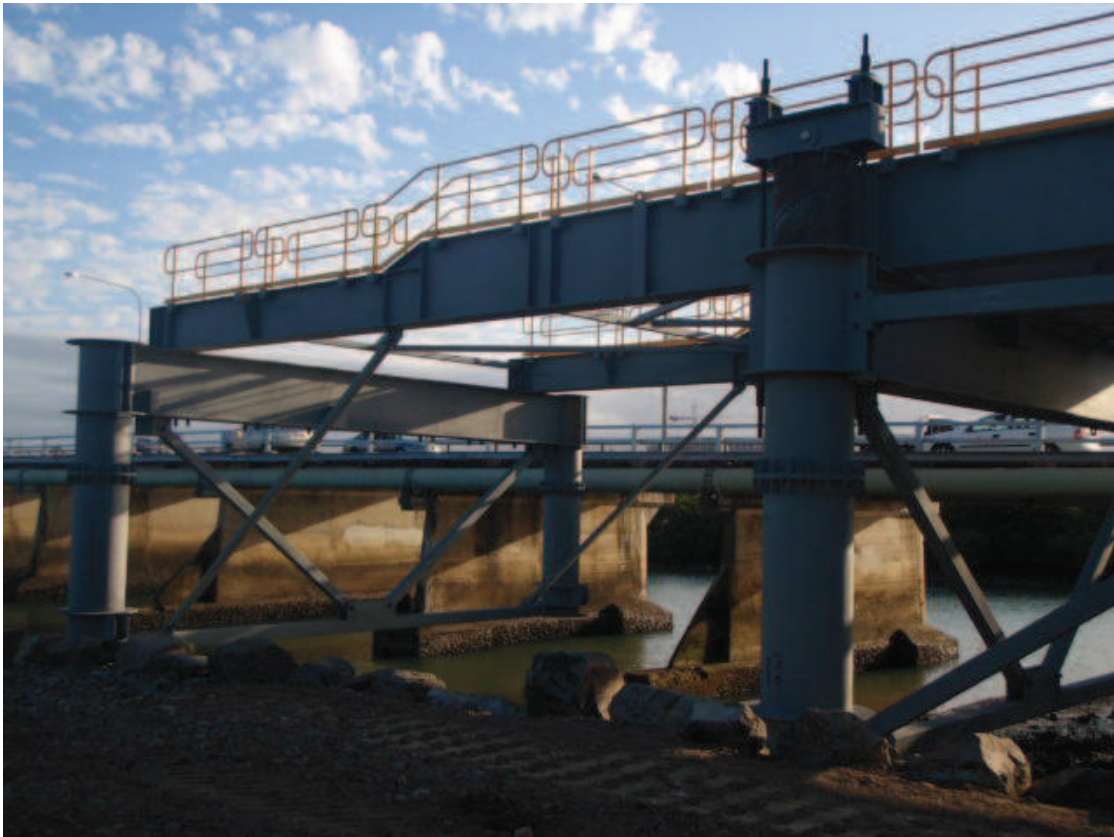
Figure 3: Example of a previous program in which piles were driven through a suspend headstock.
