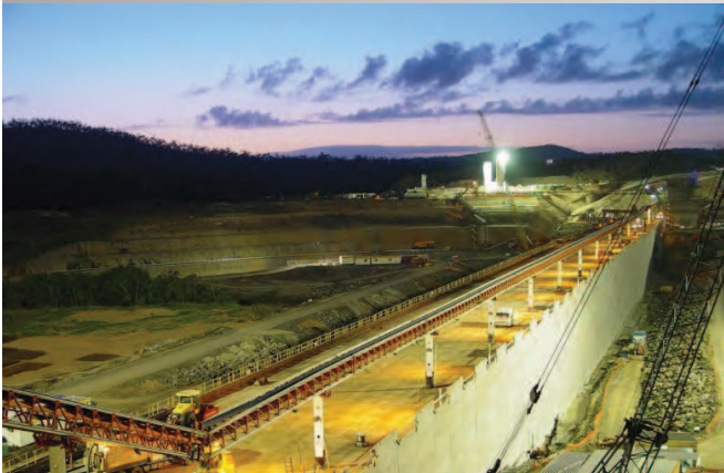
Burnett Dam – RCC Delivery Conveyor
