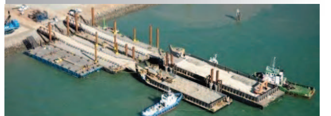
GLNG – Fisherman's Landing - Temporary RoRo Facility
