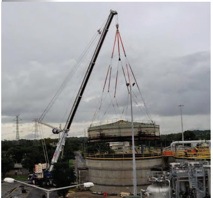
Oxley WWTP Digester Lid Retrofit
