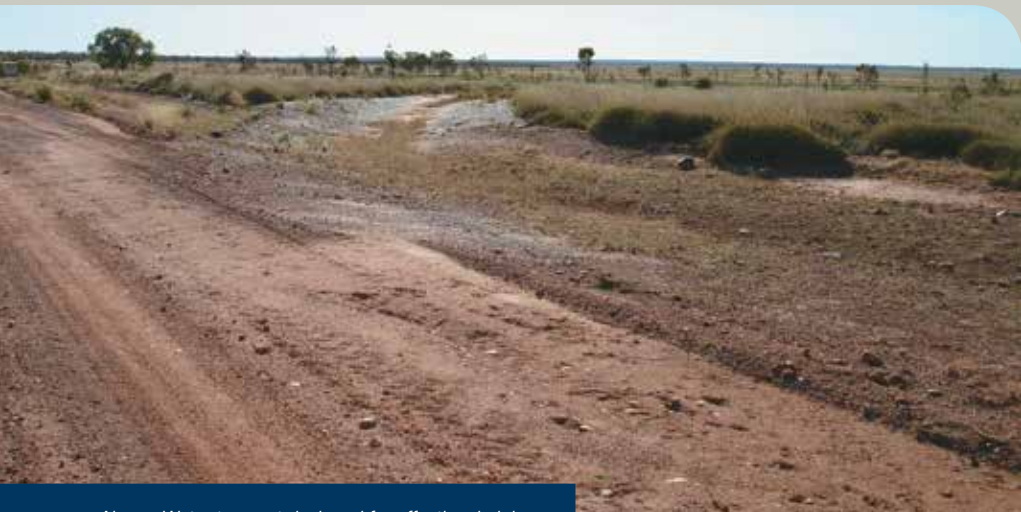
Above: Water turn-out designed for effective draining of water from a fire-break.
