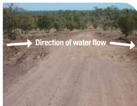
Above: A Check bank installed on a fire-break
