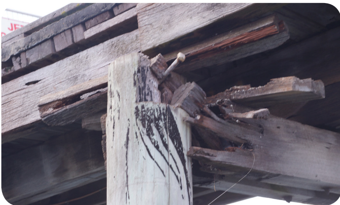
Half-cap at pile 95s.
